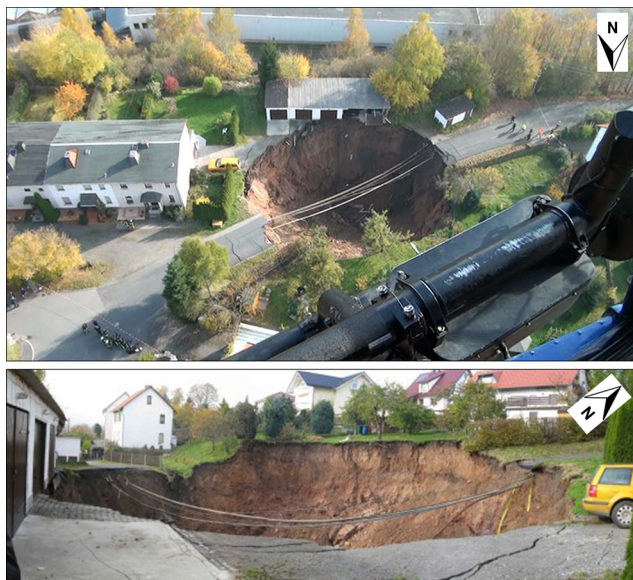
Figure 2. Photographs showing the sinkhole in Schmalkalden that opened up on 1 November 2010. It is 26 to 30 m in diameter and 12 to 17 m in depth (TLUG, 2010).
