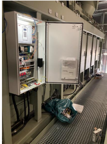
UW Wilster West: Installation des Transformatormonitorings Hitachi Energy
