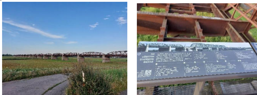
Fig 30. Kaltenhof railroad bridge monument
