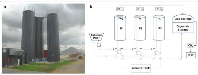
Fig. 1 Picture (a) and flow chart (b) of the sampled thermophilic biogas plant. a Left side central heating and power plant; middle the three main fermenters; right side unheated effluent tank
